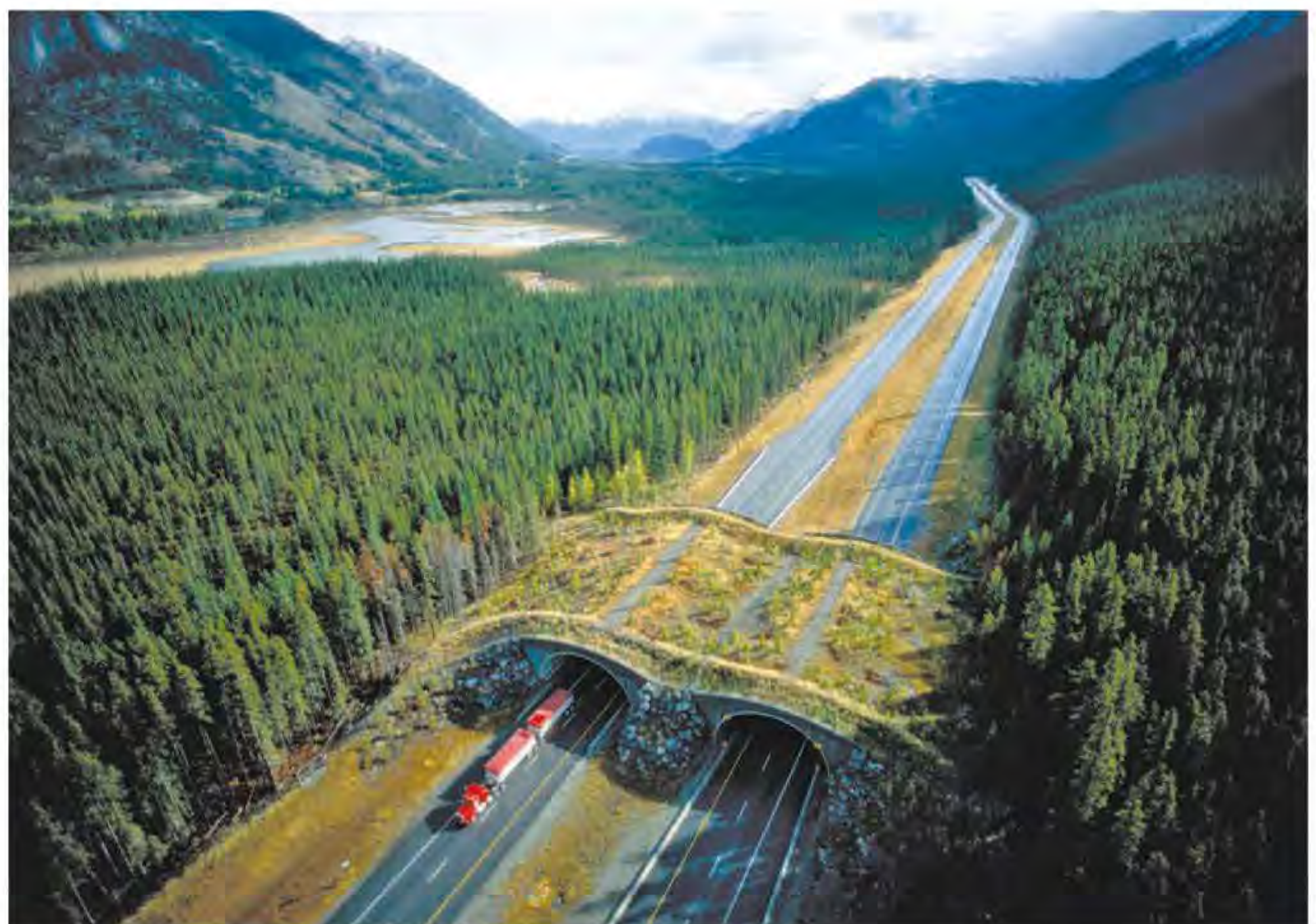
Figure 24.18 A Habitat Corridor Grizzlies and other wildlife can cross this highway overpass in Banff National Park, Canada.
